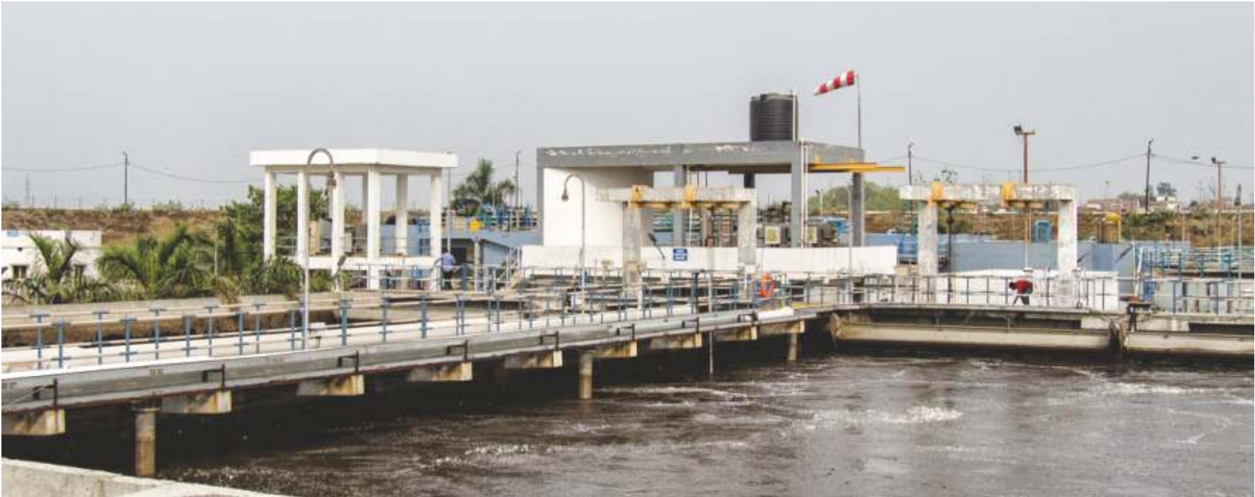
Transforming Waters, Enriching Lives: The sewage treatment plant at Naini, a testament to our commitment to a cleaner and greener future, Naini, Prayagraj
